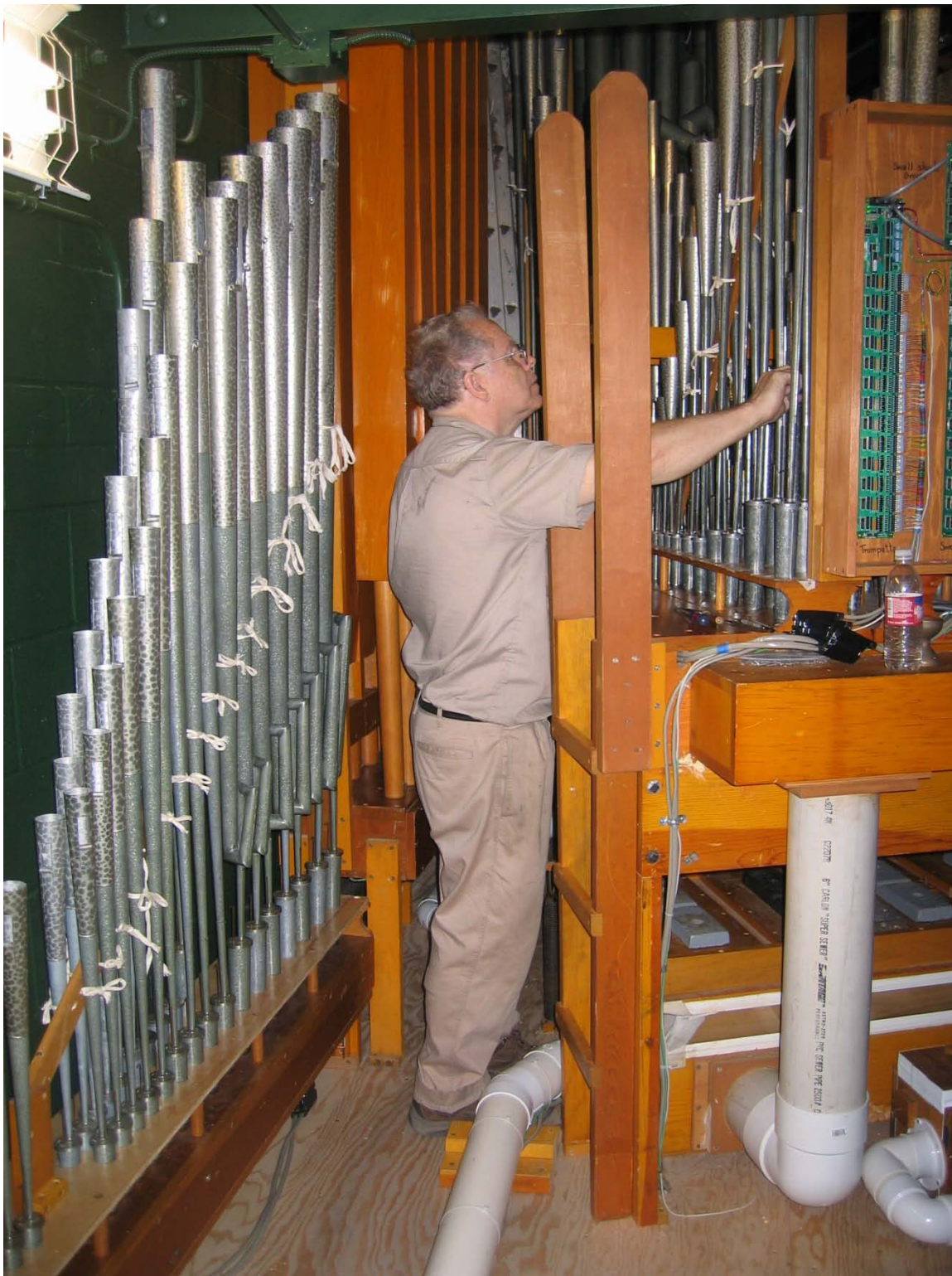
Swell chamber organ pipes in their final position—Dr. Dodrill tuning
