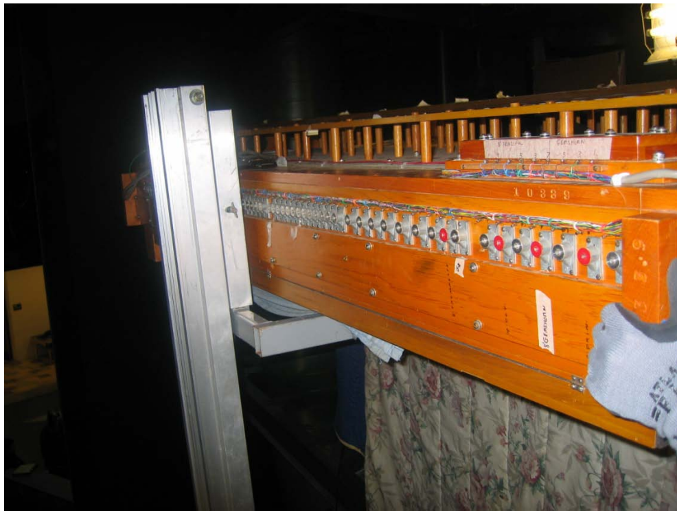
Wind chest on hand-cranked fork lift in preparation to lifting over balcony rail
